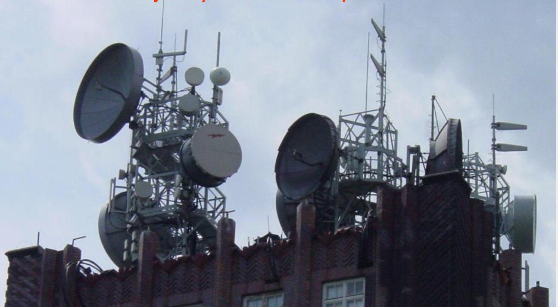
Roof of the Telecom building ( Wrocław, Poland)
